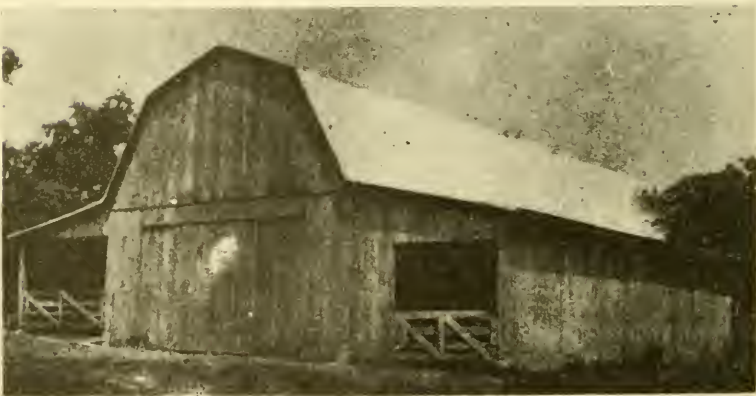
STOCK BARN AFTER REPAIR.
