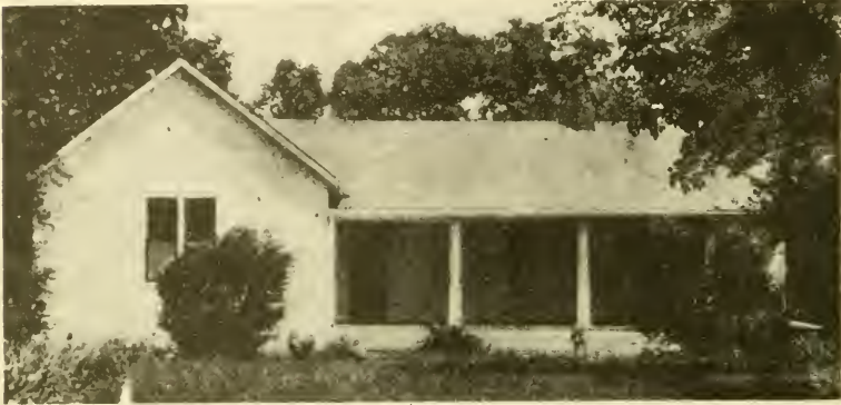
DWELLING AFTER REPAIR.
