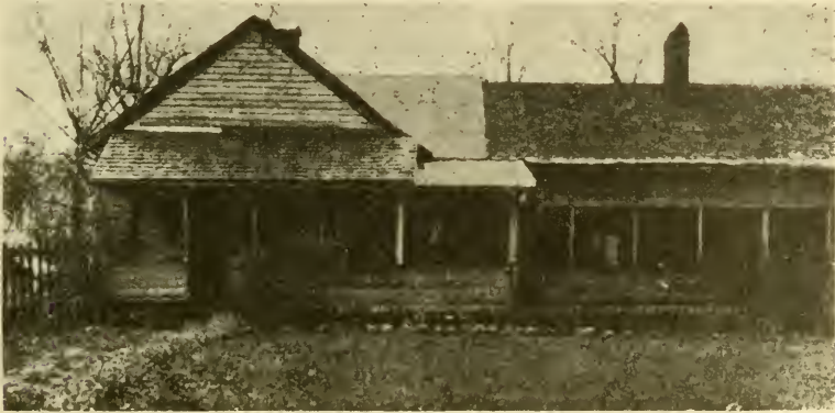
DWELLING BEFORE REPAIR. 8554X-Oglesby—370 acres—Montgomery County, Tenn.
