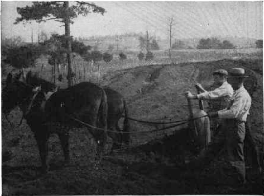
FIGURE 15.—Building up low spots in terraces and cutting down high places in the channel, before plowing, by use of team and drag-pan scraper. (Photo from Soil Conservation Service.)
